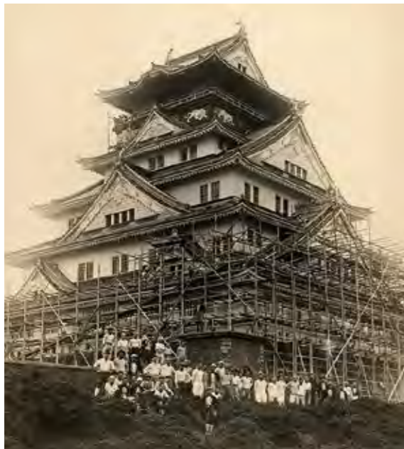
1931 The Main Tower of Osaka Castle under construction
